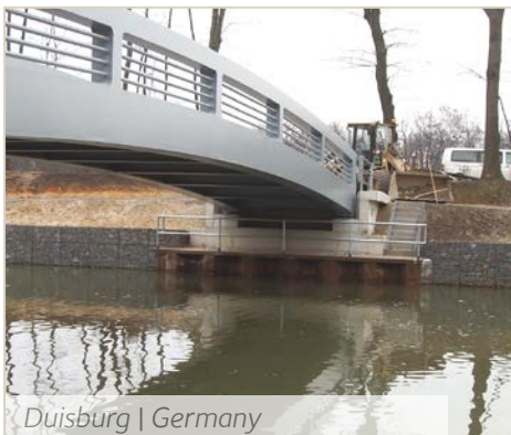
Temporary cofferdam | Germany
